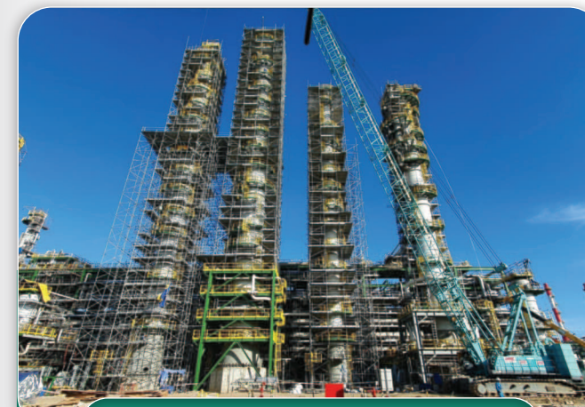
Long Son Petrochemical Complex Project
