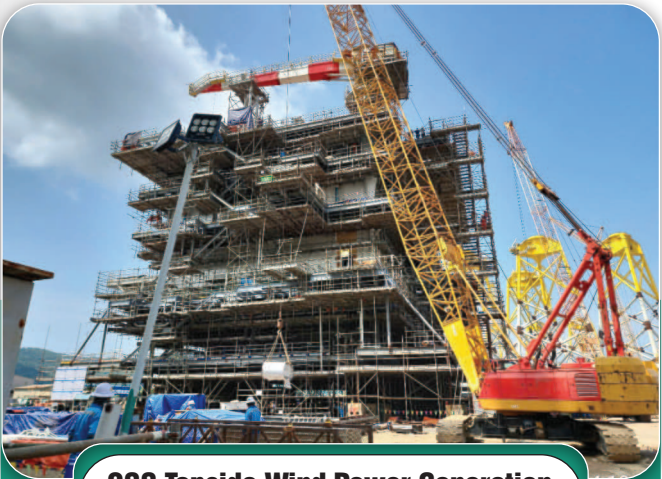
OSS Topside Wind Power Generation Project - PV Shipyard
