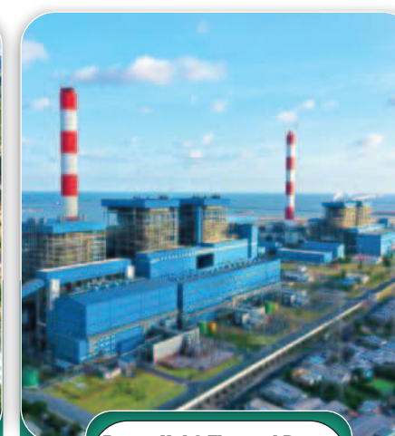
Duyen Hai 3 Thermal Power Plant Expansion Project
