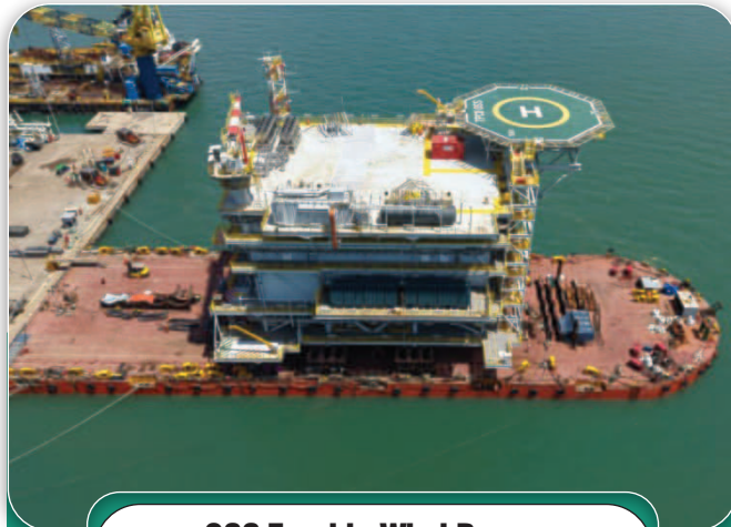
OSS Topside Wind Power Generation Project - PV Shipyard
