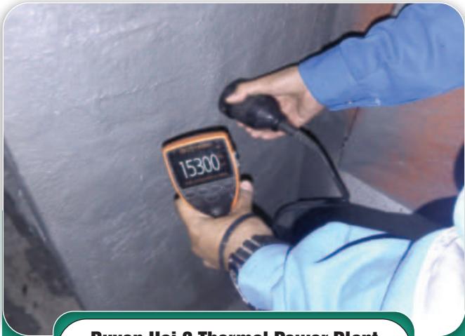
Duyen Hai 3 Thermal Power Plant Expansion Project
