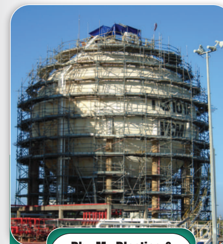
Phu My Plastics & Chemicals Plant Project
