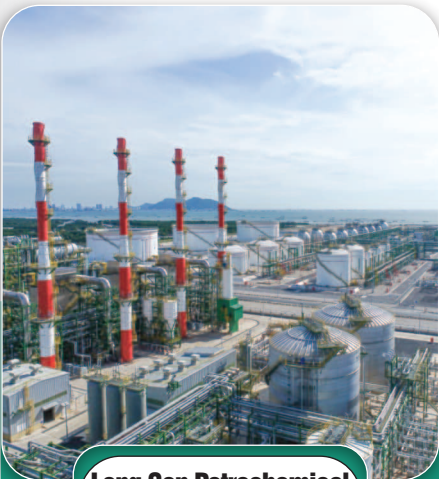
Long Son Petrochemical Complex Project
